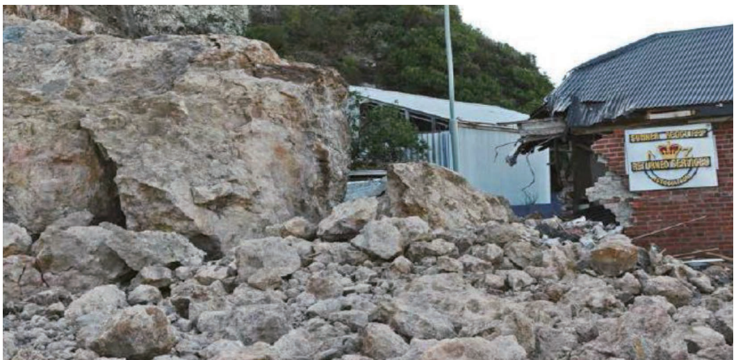
Figure 2-51: Dislodged boulders near the RSA clubrooms following the Feb 2011 Christchurch earthquake. Photo: Margaret Low, GNS Science.
